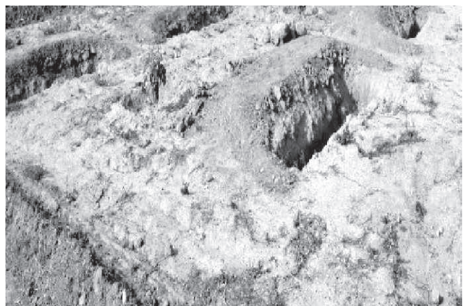
Plate-7. Contour staggered trenching
